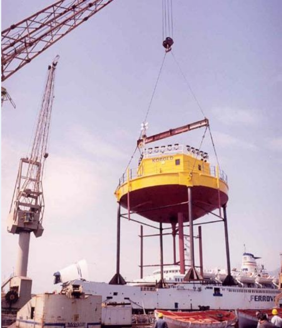
Kobold device being lifted by crane for trial deployment in the Mediterranean.
